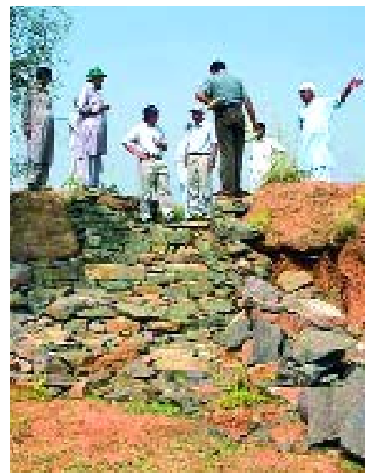
Cost-effective, simple water-regulating structures were designed by the project and implemented by farmers, for erosion control and rainwater management.
